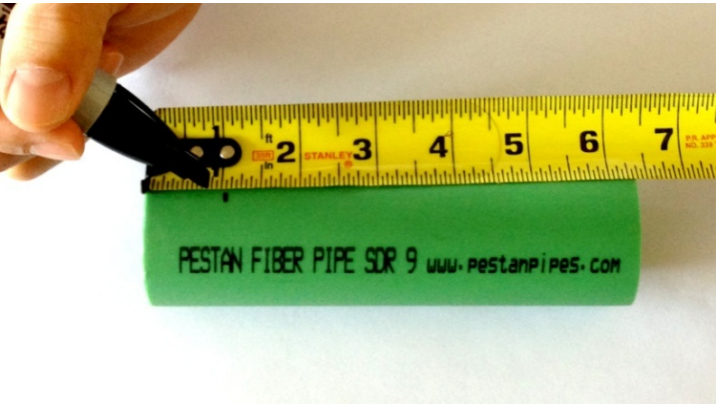
Marking pipe using measuring tape
